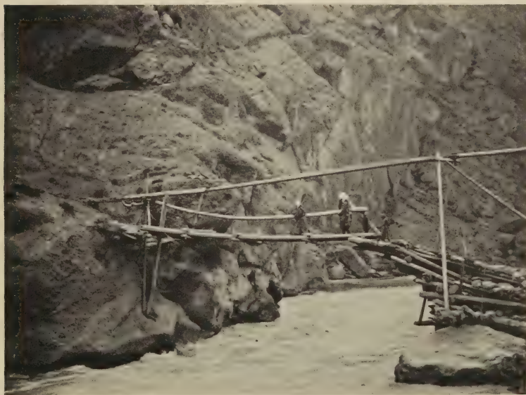
A KIRGHIZ BRIDGE BUILT ON THE CANTILEVER PRINCIPLE, KHANTEREK. THE FOREMOST OF THE LADIES CROSSING IS CARRYING TWIN BABIES
